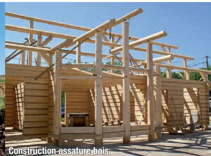
Construction ossature bois
